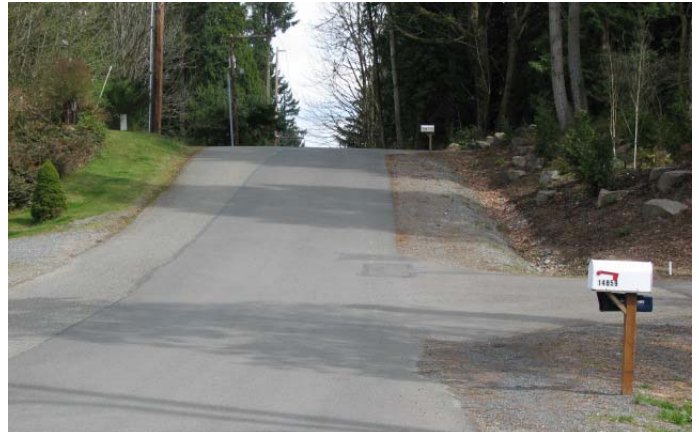
Photo 3: NE 195 th Street Inadequate Stopping Sight Distance Location
