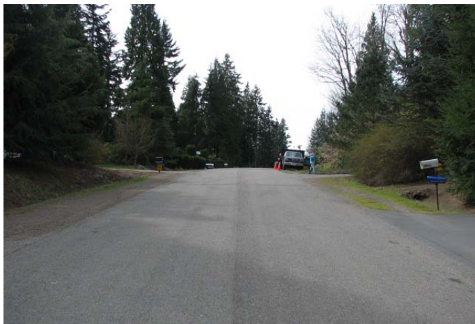
Photo 4: NE 198 th Street Looking West
